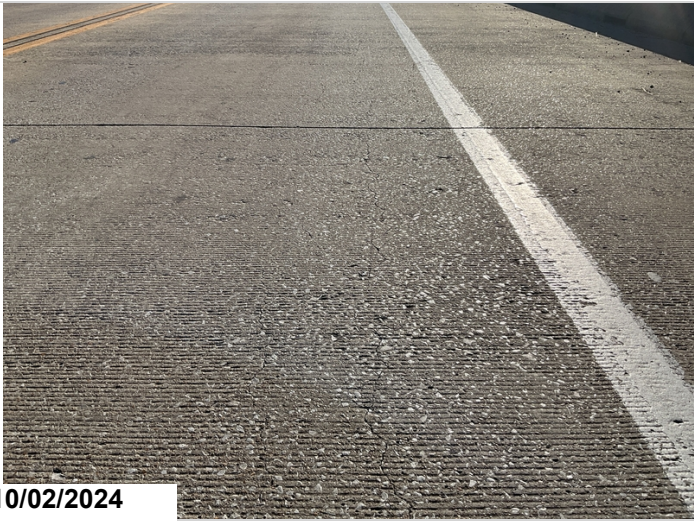
Typical moderate longitudinal cracks are present in the wheel path throughout. CS3
