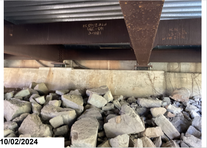
The bearings are in good condition with isolated connection issues.
