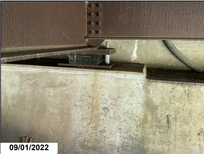
Abutment 2 at Girders 1, 2 & 5 missing one nut, Girders 3 & 4 missing both nuts. Girder 3.
