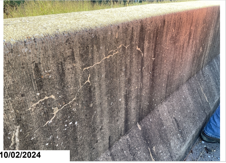
Typical railing has minor cracking, some with efflor, throughout, but is in otherwise good condition.
