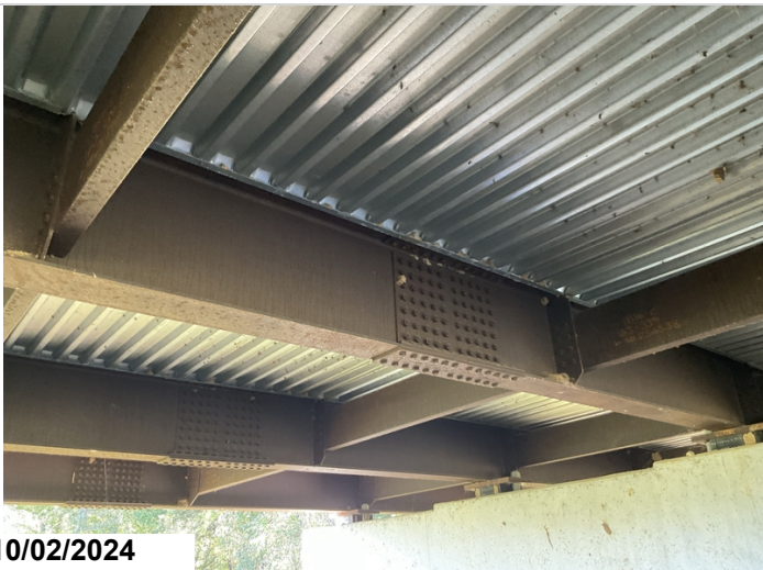
Typical splice connection
