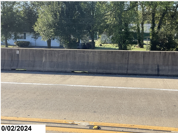
Span 4 right. 20' map cracking with efflor. CS3
