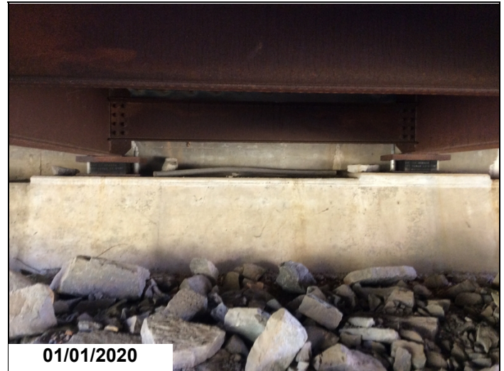
Both anchor bolt nuts are missing from Girders 3 & 4 @ Abutment 2.
