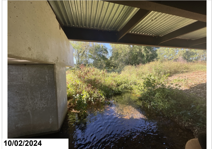
Downstream. Heavy vegetation restricting flow downstream
