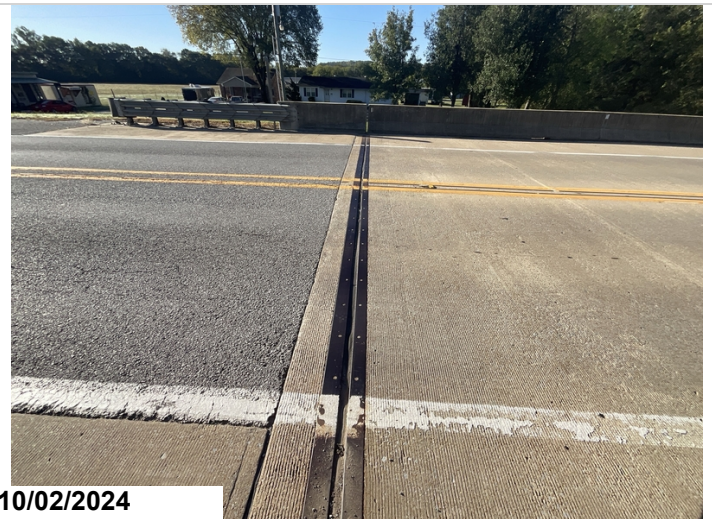
Abutment 2, joint has isolated defects throughout
