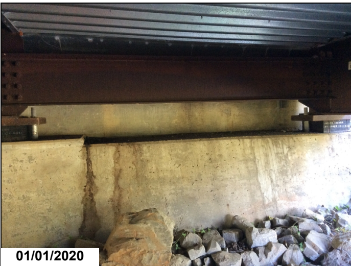
Anchor bolt nuts missing @ Girders 1 & 2 @ Abutment 1.
