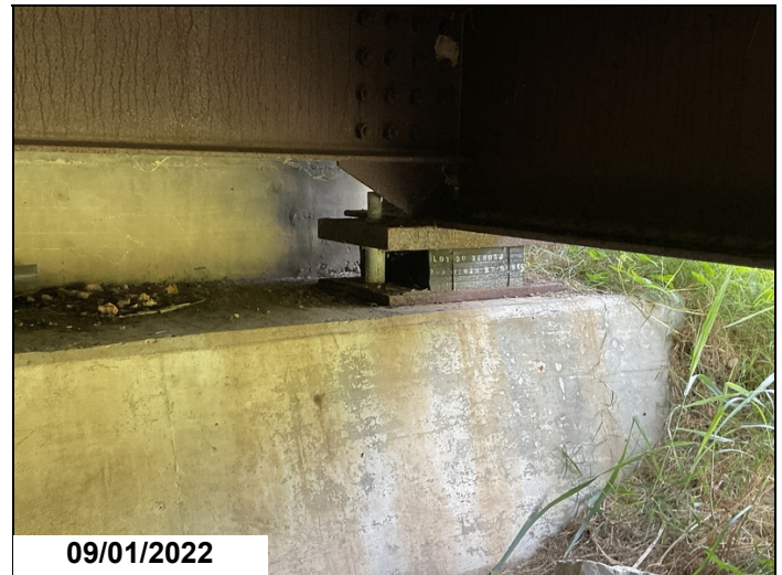
Abutment 2 at Girders 1, 2 & 5 missing one nut, Girders 3 & 4 missing both nuts. Girder 5.
