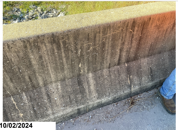
Typical railing cracks
