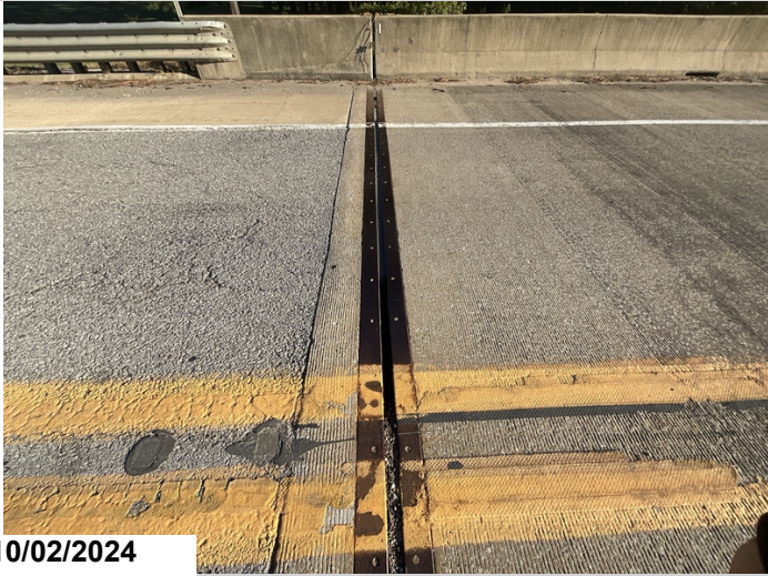
Abutment 1, joint: has adhesion loss for in the center line and left shoulder. 4LF CS4
