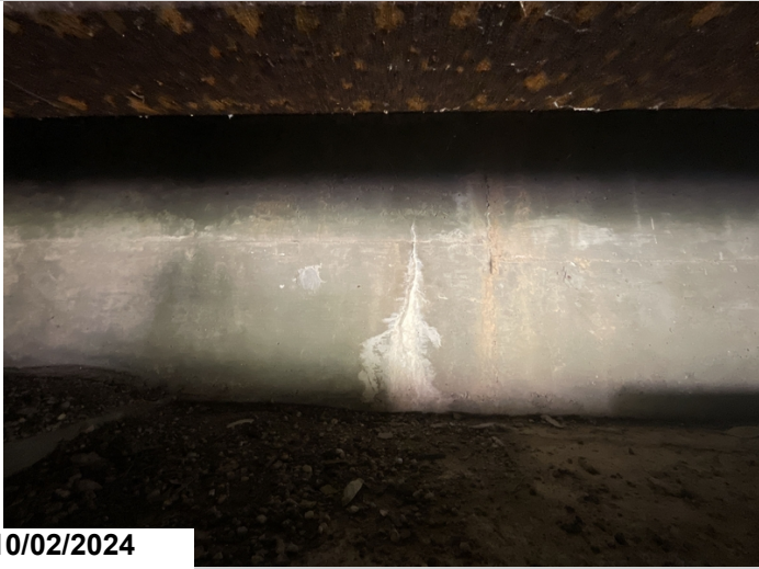
Abutment 2, backwall: has efflor cracks with buildup. 4LF CS3
