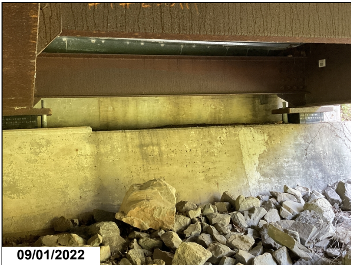
Anchor Bolt Nuts Missing Abutment 1 at Girders 1 & 2 missing one nut.
