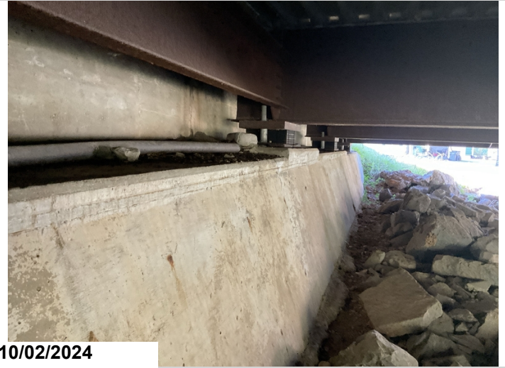
Abutment 2, bearings, are missing anchor nuts. 5EA CS2
