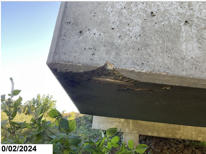
Bent 3, left: spall. CS2
